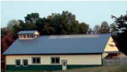
Loading and Handling Facility
